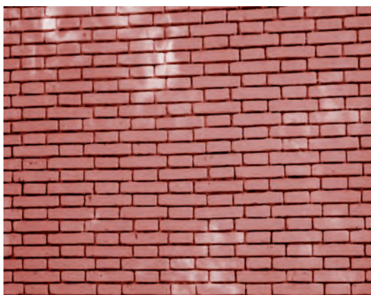
(a) Brick wall
