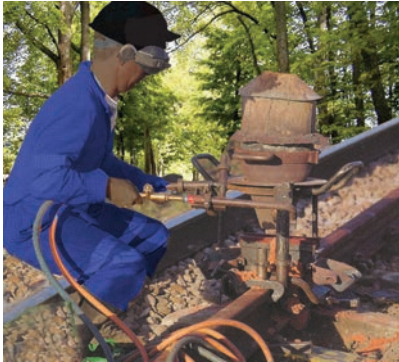
Figure 3.11 Thermit process for joining railway tracks
