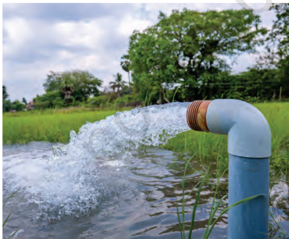
Fig. 1.15. Extraction of groundwater
