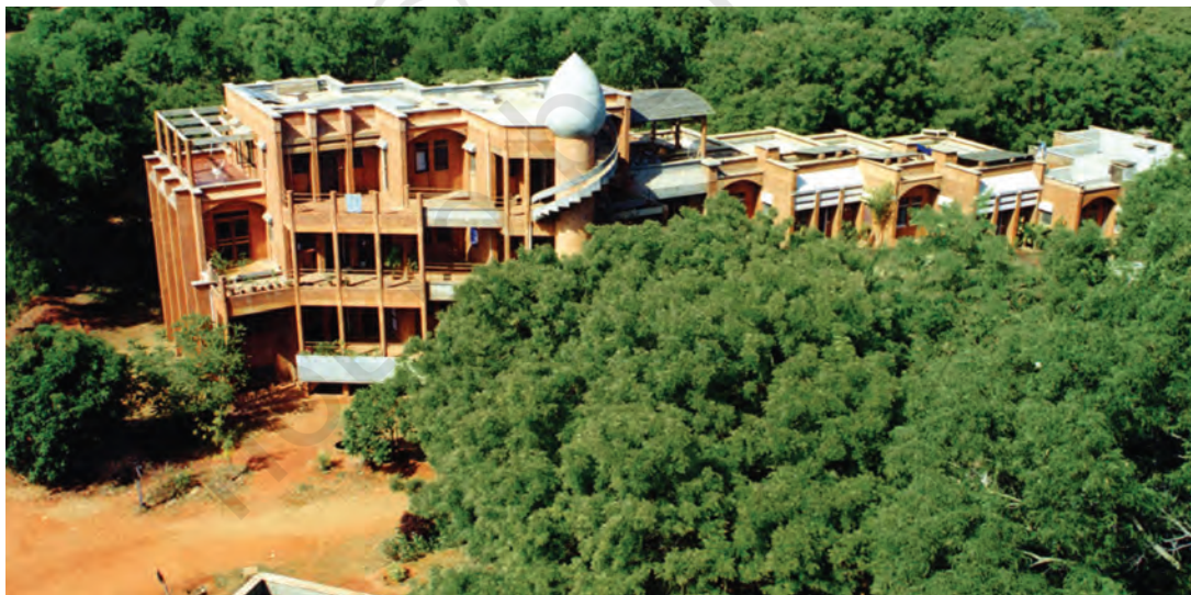
Fig. 1.19. A community building in Auroville constructed by Auroville Earth Institute (which holds the UNESCO Chair for Earthen Architecture). This modern building is made of mud using special techniques.
