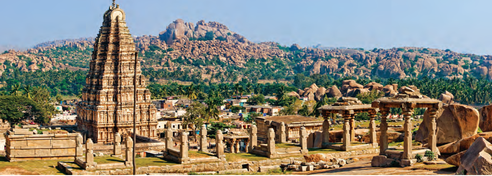
Fig. 2.11. A section of the ruins of Vijayanagara city (present-day Hampi). The large building is the Virūpākṣha temple.
