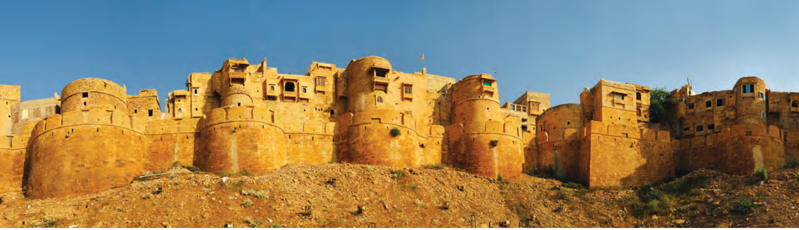
Fig. 1.18. Jaisalmer fort, Rajasthan. A mud structure built in the 12 th century and refurbished later using sandstone.
