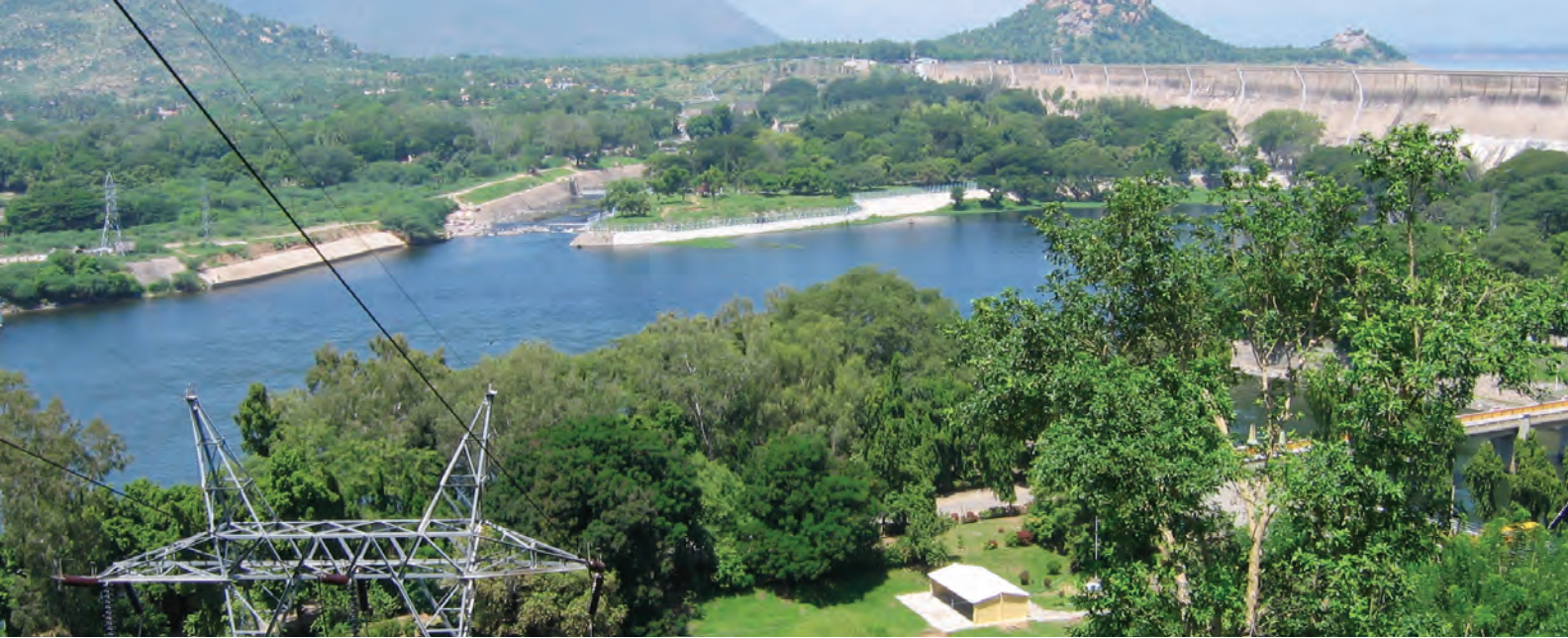
Fig. 1.13. Mettur dam in Tamil Nadu built on the Kaveri river
